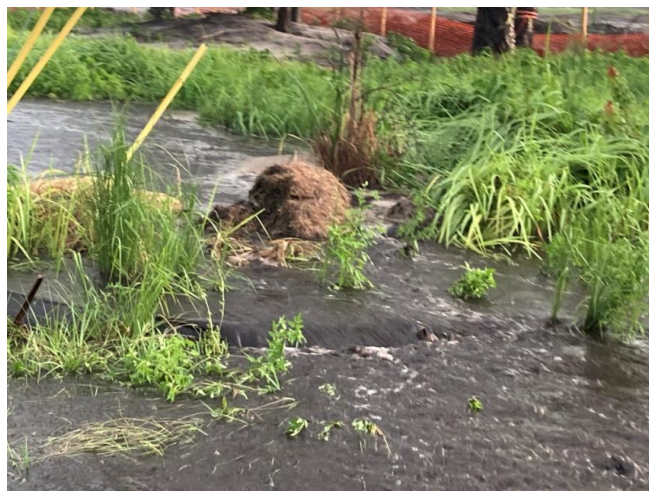
b. Turbid water discharging from construction site following 2.5-inch rainfall on 8/10/20
