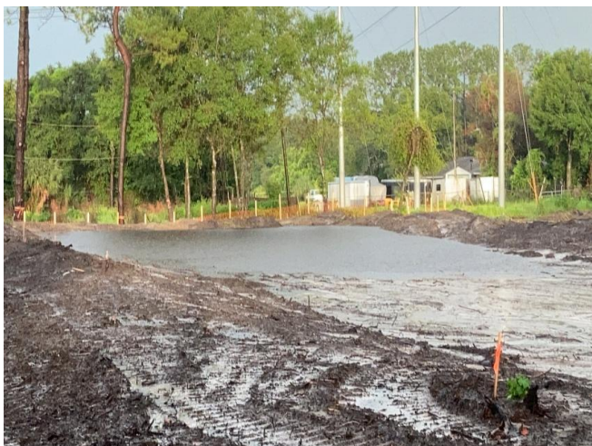
a. Temporary stormwater pond on construction site.
