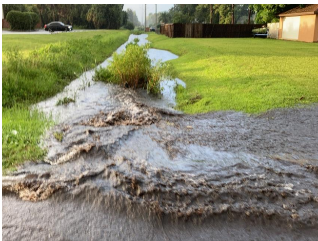
c. Water flowing through channel along powerline on 8/10/20
