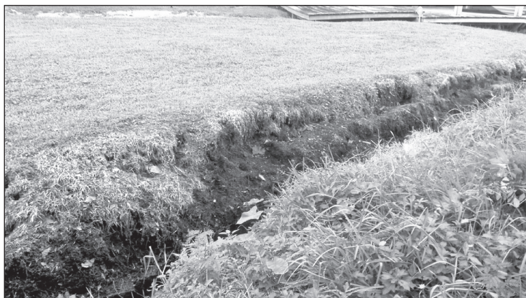
Wash out of Playa Way Drainage Ditch November 2019
