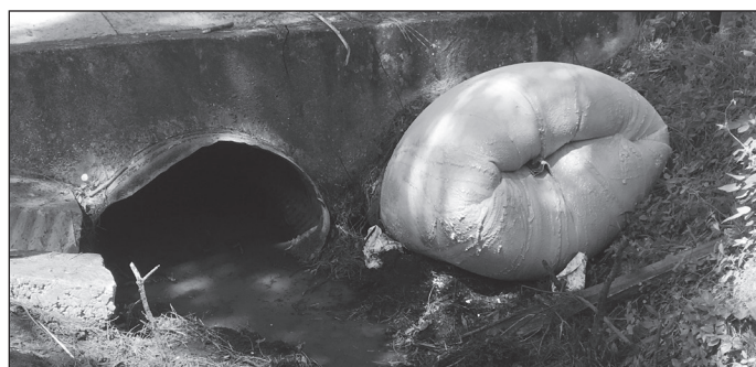
Collapsed pipes were causing road depressions and blockage on Bear Lake Circle. Seminole County reinforced the stormwater pipes under the road late September 2019 with fiberglass sleeves. The pipes were cleaned and fiberglass material inserted into pipe, cooked from 120 to 180 degrees, sealing and reshaping the collapsed pipes. This system is used as an emergency bypass between Bear Lake and Little Bear Lake. Did you know there once was a canal between the two lakes?
