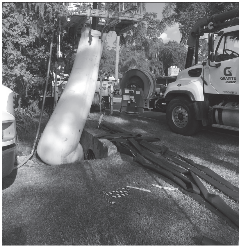
Collapsed pipes were causing road depressions and blockage on Bear Lake Circle. Seminole County reinforced the stormwater pipes under the road late September 2019 with fiberglass sleeves. The pipes were cleaned and fiberglass material inserted into pipe, cooked from 120 to 180 degrees, sealing and reshaping the collapsed pipes. This system is used as an emergency bypass between Bear Lake and Little Bear Lake. Did you know there once was a canal between the two lakes?
