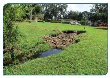
Lake Asher storm water, mud and debris flushed out to Bear Lake during Hurricane Irma after drain collapsed.
