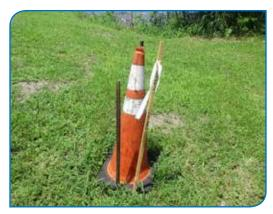
Prior to the rains from Hurricane Irma, the cone marks a sunken void of soil under the grass and over the broken storm water pipe on July 25, 2017 after 40" of rains in June & July.
