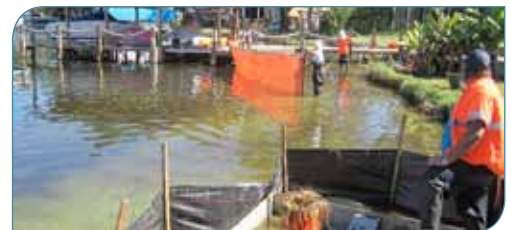
The area around the drain is cleared until North cold front winds send endless floating eelgrass back again.
